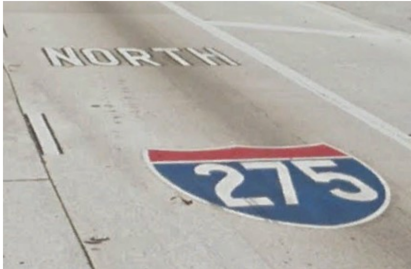
Figure 4.2-4. Cardinal Direction Markings
