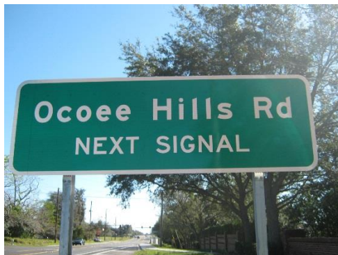
Figure 2.37-1. Advance Street Name Sign at Signalized Locations
