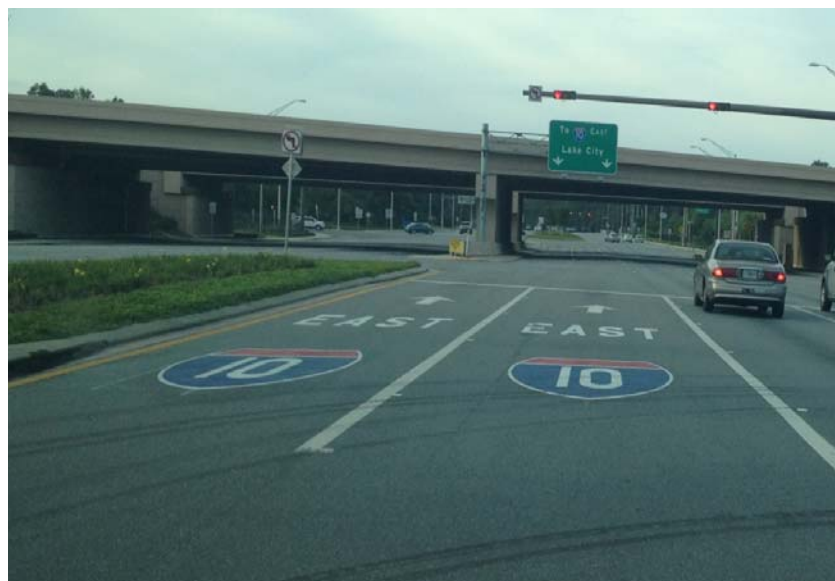
Figure 4.2-7. Pavement Markings for Wrong Way Treatment
