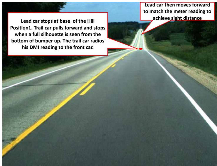
Figure 3. Sag Vertical Curve
